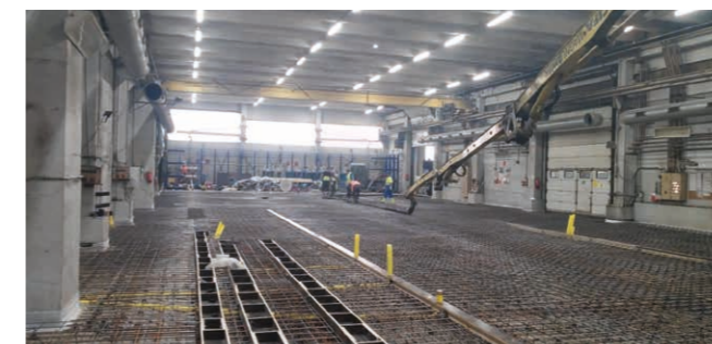
Reinforcement of hall floor and layout of the rail system for the lifting and rotating equipment
