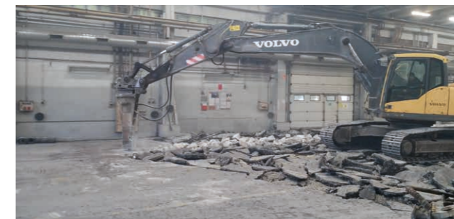
The existing hall floor is taken up
